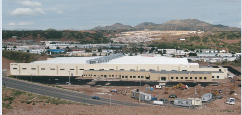
Belden's Mexico new facility
